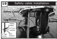
Fan and light kit combinations over 70 lbs, in both flush and downrod mode the safety cable must be installed into the house structure beams using the 3" lag screws,washers, and lock washers. provided. Make sure that when the safety cable is fully extended the lead wires are longer than the cable and no stress is placed on the lead wires.
